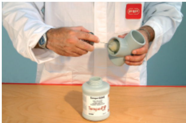
Photo 8-9-10: Applying the "TemperGLUE" solvent cement
