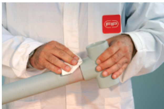
Photo 12: Removal of cement excess
